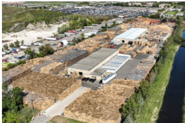
Overhead photo of Taylor, MI Facility
